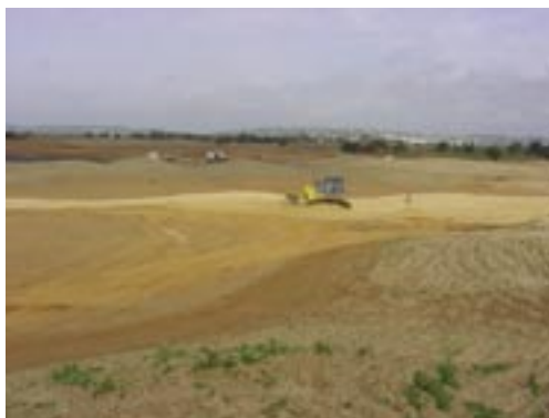
Figura 3.3-23 Bulldozer a distribuir top-soil num fairway
